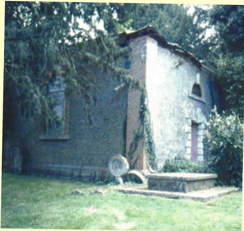
Heathcote mausoleum before restoration
