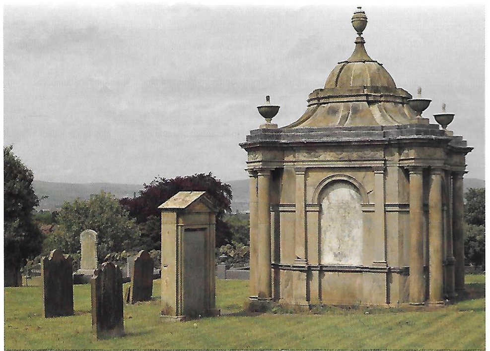
The Greg Mausoleum in the cemetery. It was probably designed by Roger Mulholland, and its brick core is rendered and detailed with cut stone. It has recently been restored
