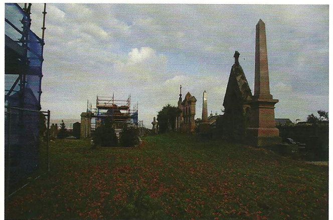
Work on Greg and Rainey proceeds.
